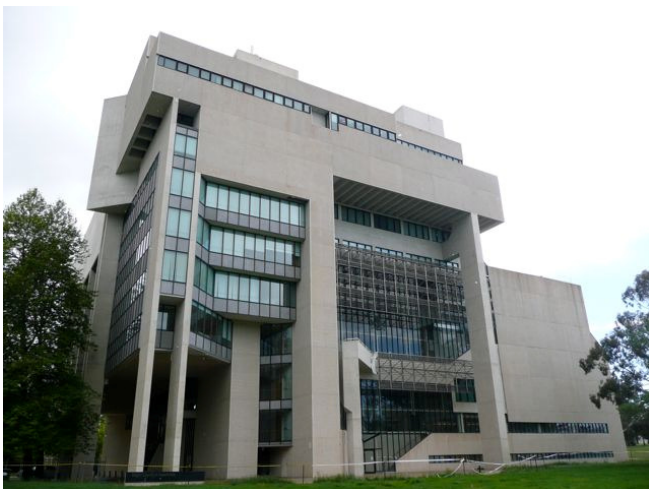
Figure 7. High Court from the lake-side Source: Duncan Marshall
